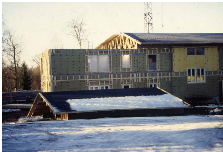
Figure 8.13 Roof used as weather protection during erection of the structure
